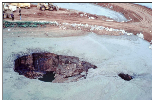
Figure 3 This post-collapse view of the West Plains Lagoon shows two sinkholes that developed as the lagoon drained.
