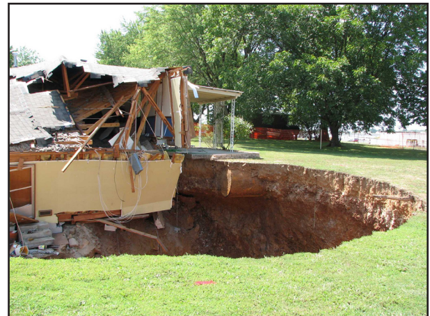
Figure 12 The collapse structure developed in a structured reddish-brown, cherty, and clayey residuum as can be seen from this view. From the angle of this picture the lack of subsidence of the area is apparent. Also visible is an abandoned steel septic tank.
