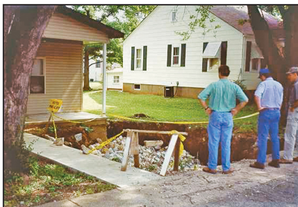
Figure 5A Collapse in residential neighborhood, Farmington, Missouri. This collapse had been repaired with soil fill only, but it reactivated.
